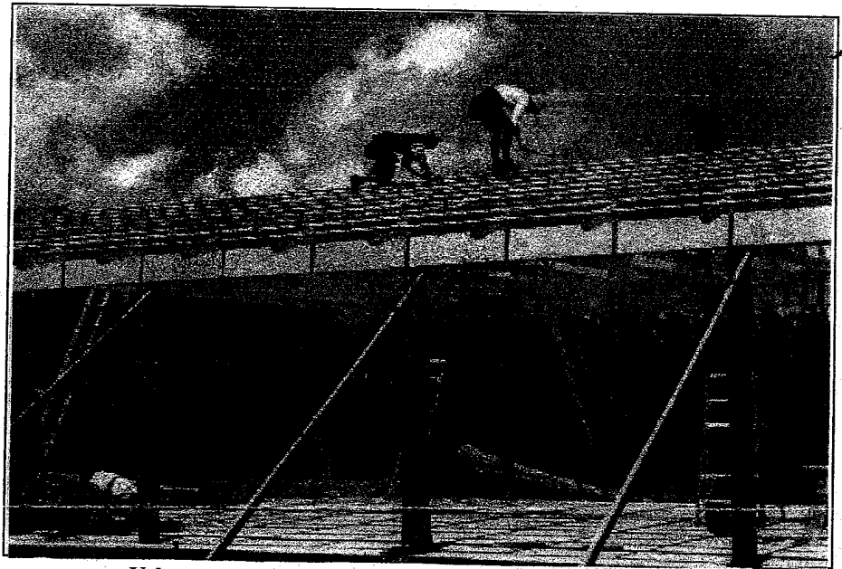
Volunteers work on the roof of Seaview's new park pavilion.
